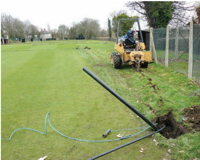
Insetting the channels of the pipework around the lawns
