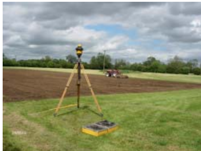
Preparation of the courts showing laser levelling equipment, with receptor above grader behind tractor which receives instructions.
